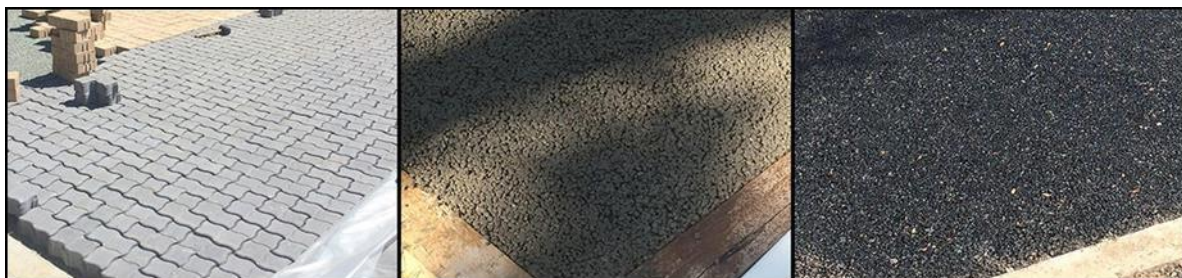
Figure 4: Examples of materials used in permeable paving (from left to right) permeable interlocking pavers, permeable concrete and pervious asphalt
